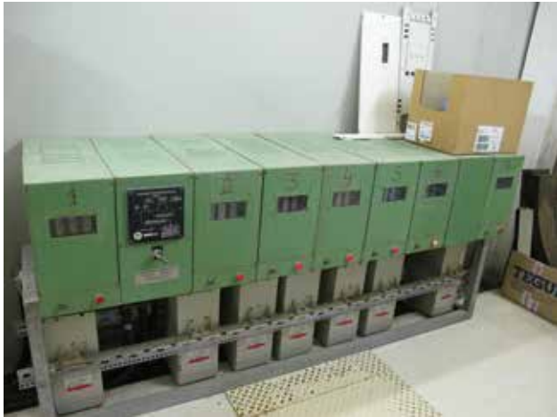
Figure 22. Capacitor batteries.
